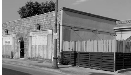
Remove barriers and add lighting to activate existing outdoor dining spaces
