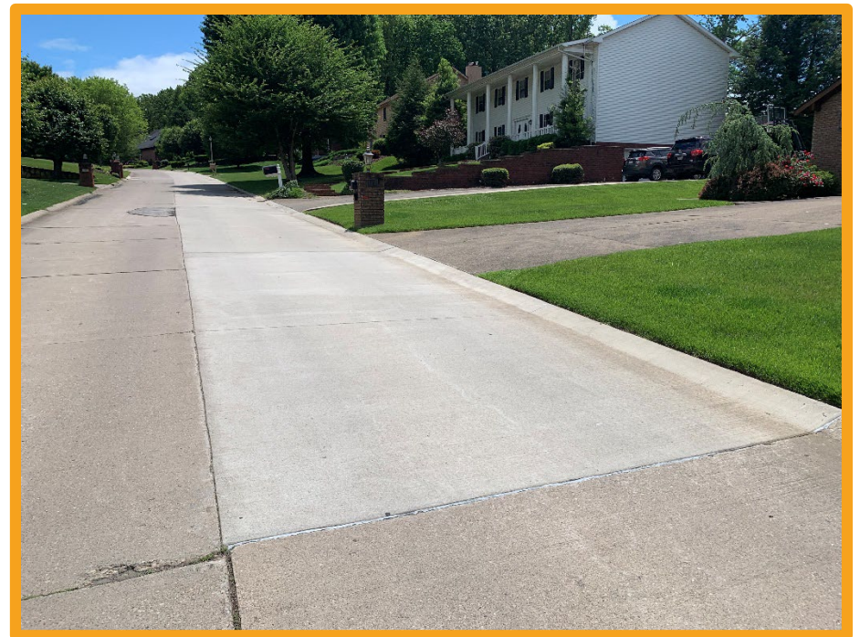
Stamford Park Dr. road repair
