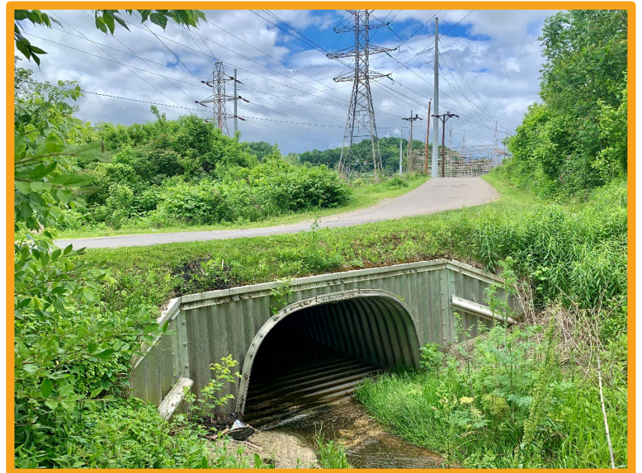
Nickel Plate Rd. culvert replacement
