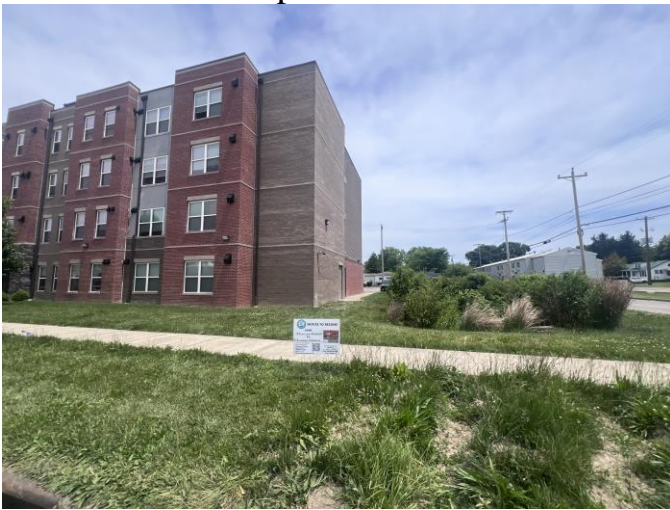
View of the southwest corner of the block at the corner of 10 th Street West and 5 th Avenue West.
