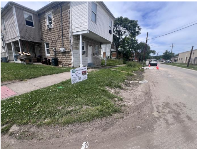
View of the southeast corner of the block at the corner of 9 th Street West and 5 th Avenue West.
