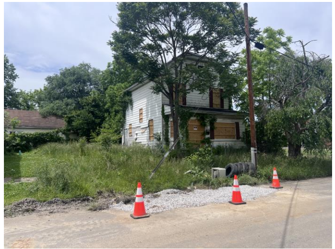
View of the boarded up property at 522 9 th Street West.
