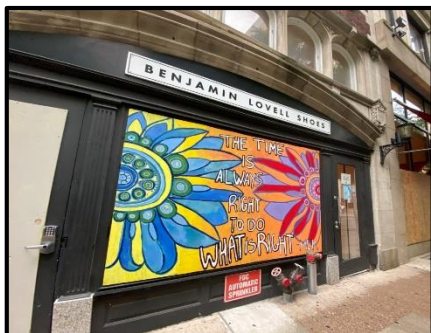
Painting boards on vacant properties
