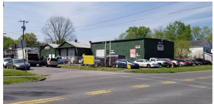
Location of Bishops Auto on the corner of 8 th Avenue and 23 rd Street.
