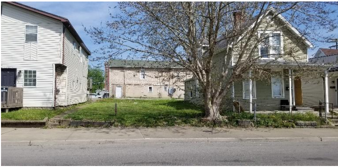
View from the street, looking north at 1842 7 th Avenue.
