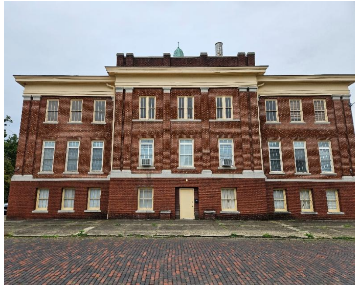
View of property looking south from Jefferson Avenue.
