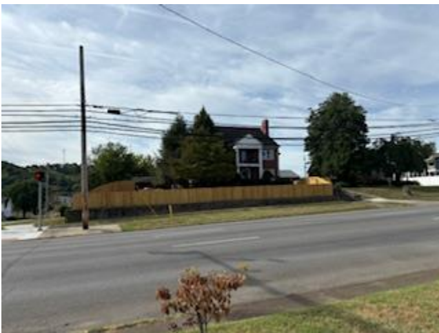
View of privacy fencing looking south from across 3 rd Avenue.
