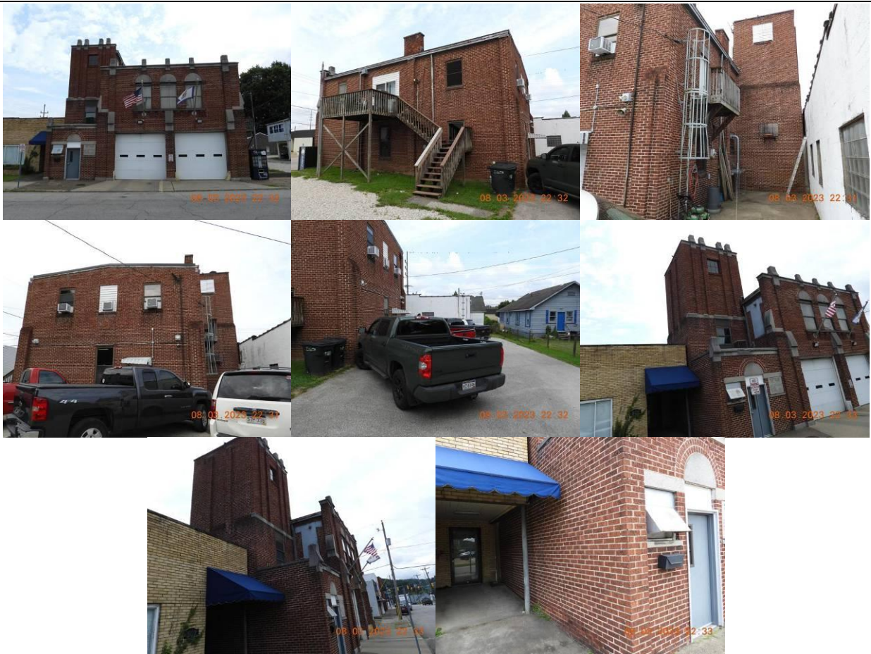
Typical exterior views of the subject property's improvements.
