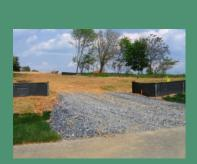
CONSTRUCTION EXIT SHOULD BE NO LESS THAN 70 FEET (EXCEPT ON A SINGLE RESIDENCE LOT WHERE A 30 FOOT MINIMUM LENGTH WOULD APPLY). WIDTH SHOULD BE A MINIMUM OF 10 FEET AND THE THICKNESS SHOULD BE 6 INCHES DEPTH. GEOTEXTILE FABRIC SHALL BE PLACED OVER THE ENTIRE AREA PRIOR TO THE PLACING OF STONE
