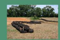
SEDIMENT TRAPPING DEVICE LIKE WATTLE, EROSION EEL, OR SILT FENCE SHALL BE CONSTRUCTED AS ONE OF THE FIRST STEPS IN GRADING. THESE NEED TO BE INSPECTED AFTER RAIN EVENTS OR EVERY WEEK. SEDIMENT SHOULD BE REMOVED WHEN IT REACHES 50 % OF THE FENCE.
