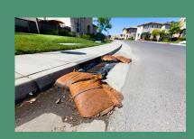
STORM DRAIN INLETS SHALL BE PROTECTED DURING CONSTRUCTION. INLETS SHOULD BE INSPECTED WEEKLY AT A MINIMUM AND DAILY DURING STORM EVENTS. INLET PROTECTION DEVICES SHOULD BE CLEANED OR REMOVED AND REPLACED BEFORE SIX INCHES OF SEDIMENT CAN ACCUMULATE.
