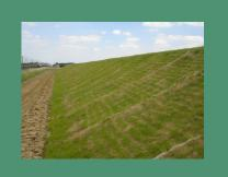
VEGETATION CONTROLS EROSION BY REDUCING THE VELOCITY AND THE VOLUME (BY INCREASING INFILTRATION) OF OVER LAND FLOWS. SOIL STOCKPILES MUST BE STABILIZED AND PROTECTED ALSO. ALL GRADED AREAS THAT ARE AT FINAL GRADE MUST BE SEEDED AND MULCHED WITHIN 7 DAYS.
